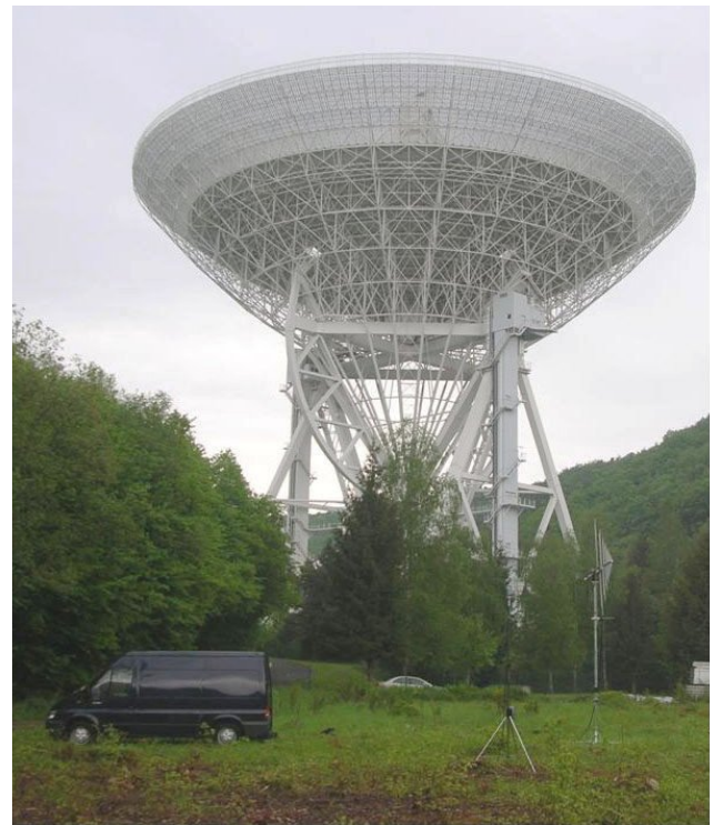
Fig. 9. ASTRON equipment to measure low frequency RFI is placed at the Effelsberg LOFAR site.
